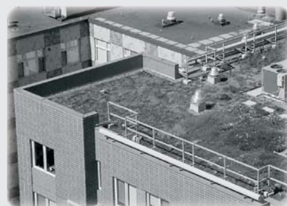
Photo: City of Portland Housing Authority
